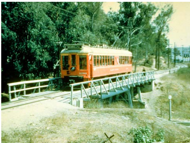
SANTA MONICA AIR LINE CROSSES OVER MOTOR AVENUE
