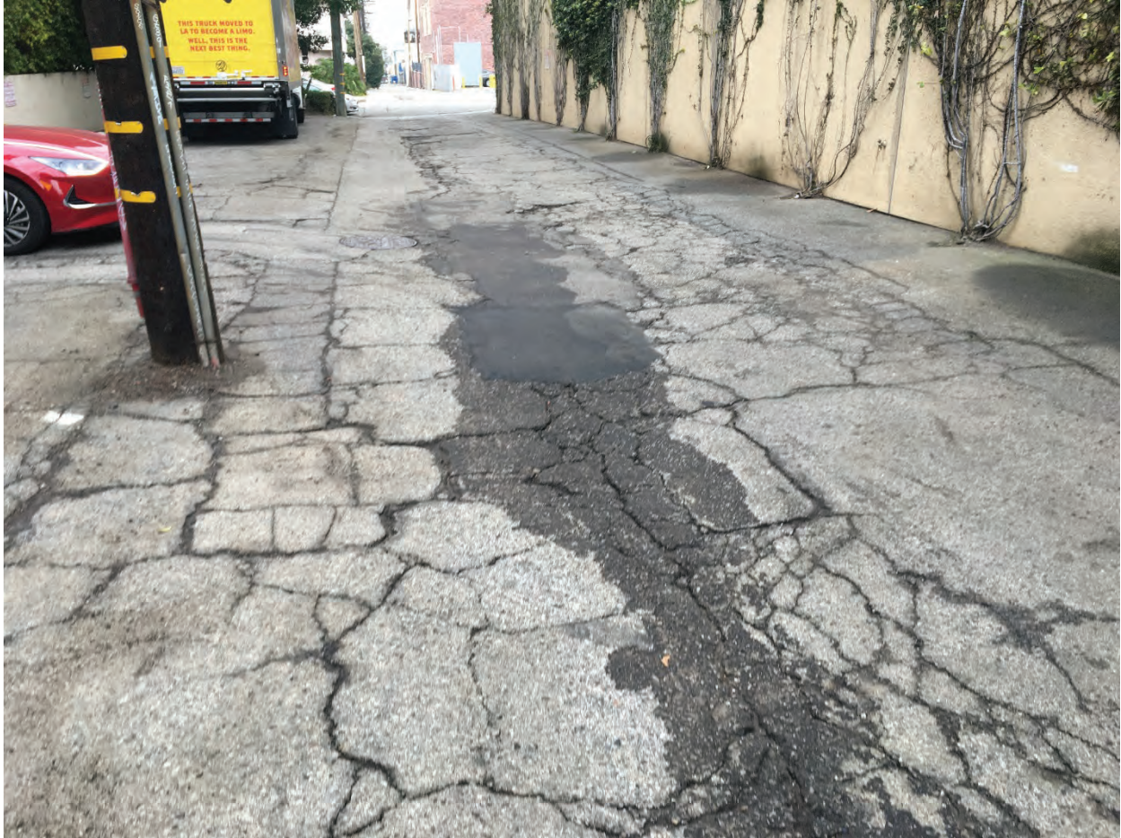
Figure 4. Shows areal extent of leaked fluid migration
